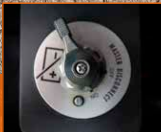
Battery cut-off switch
