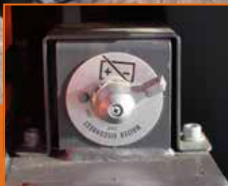
Battery cut-off switch
