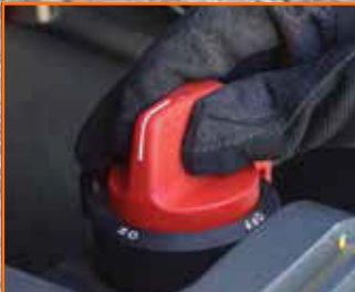
Battery cut-off switch
